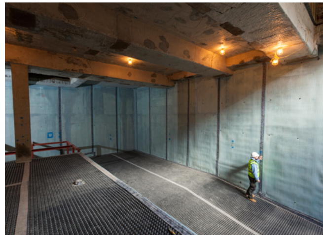
Platon P8 was fixed to the walls with deeper studded Platon P20 laid to the floor
