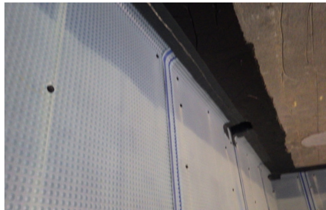
Lower basement level showing Platon P8 membrane on wall to soffit detail sealed with TT Vapour Membrane. 40mm discharge outlets drain down from the level above and angle back towards perimeter liner wall.
