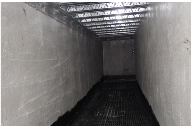
Completed trench looking up to suspended steel floor to lower level basement.
