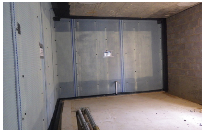
Upper basement level showing P8 membrane to walls and banded perimeter drainage channel.
