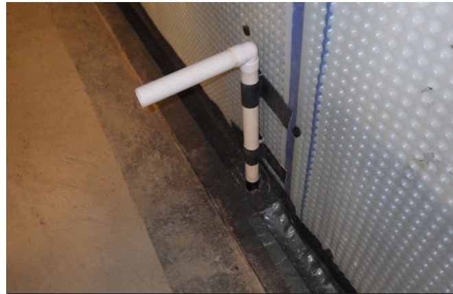
Platon P8 membrane to wall at upper basement level with perimeter drainage channel sealed with TT Vapour Membrane and Corner Strip, showing access point via 40mm pipe and 90° bend.
