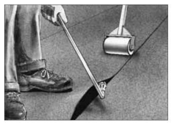
**Method B:** Unroll the full length of the felt, stretch and place in correct position. Complete the mechanical fixing of the felt. Join the overlap by inserting a gas burner between the two sheets. Direct and move the burner backwards and follow immediately with a roller pressing the overlap together. Ensure that the full 12 cm width of overlap is torched.
