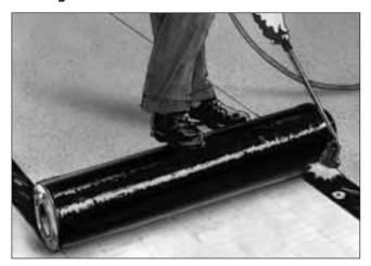
**Method A:** Unroll the full length of the felt, stretch and put in correct position, reroll the felt on a hard core. Weld with a gas burner in front of the roll while unrolling.
