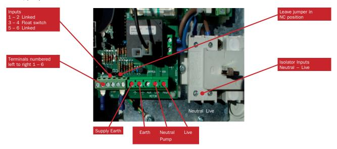
The panel is designed to control a single pump from a single float switch. An optional high level alarm float may be installed, set above the pump float, to warn of excessive water level.
