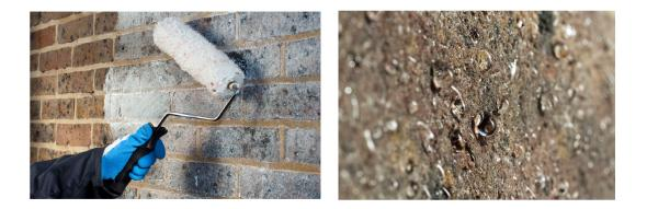
**Triton TRIPROOF CREAM** is an odourless water repellent treatment for masonry walls forming a water repellent barrier. It is formulated from a blend of silanes and siloxanes which line the pores of the masonry walls to from a water repellent matrix. The **Triton TRIPROOF CREAM** once applied allows the walls to breathe whilst protecting them from further damp penetration.
