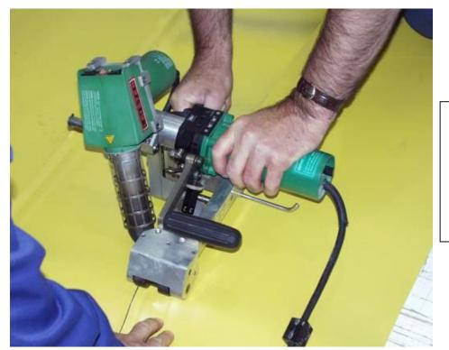
Heat welding with automatic welding machines (double seam) – welded seams as strong as the membrane
