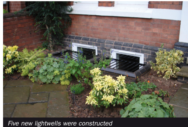
Five new lightwells were constructed
