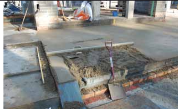
Triton SBR latex admixture was added to the initial screed
