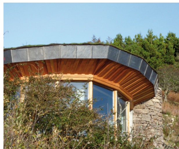
There are far reaching sea views from windows tucked beneath the extensive turf roof construction
