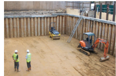
Watertight Concrete Basement in Construction
