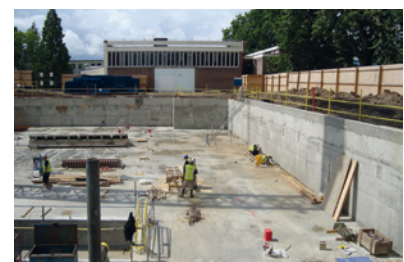
Type B Waterproofing
