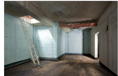
Existing Basement Waterproofing
