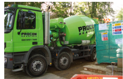
Waterproofing Concrete Structures Below Ground
