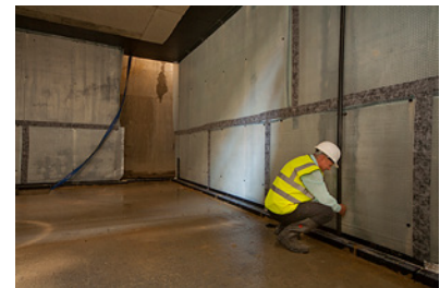
New Build Basement Waterproofing
