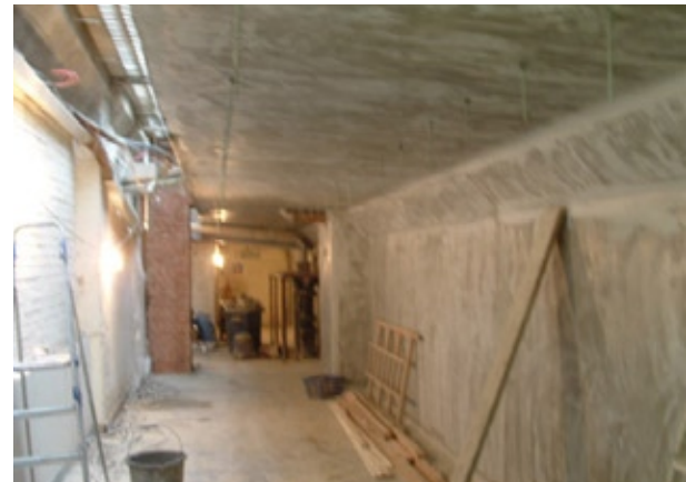
After the installation of the T55 tanking system, before painting
