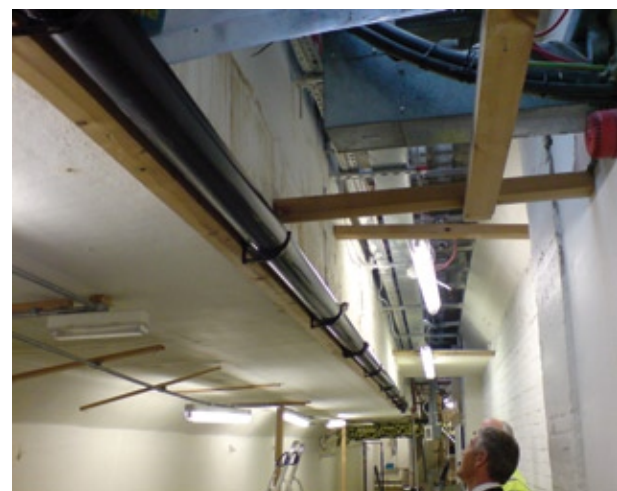
Temporary guttering system in place
