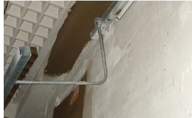
Patch repairs with 3:1 sand cement render
