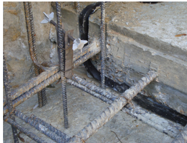
Sealed construction joint
